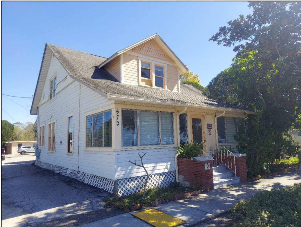
Front house of the Rental Property
